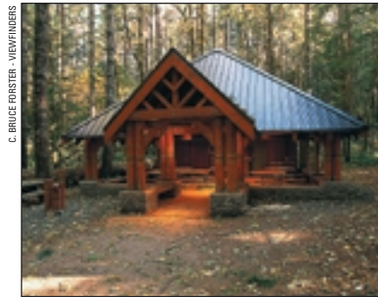
Enjoy a unique look into the life of fish at the Cascade Stream Watch off of Hwy 26 at Welches. See stream-life in action with a direct look into the stream through a special glass display.
